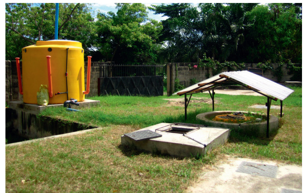
Lumbrifilter and Daphniafilter (covered)
