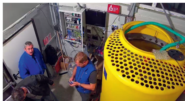
Biofilter room with lumbrifilter
