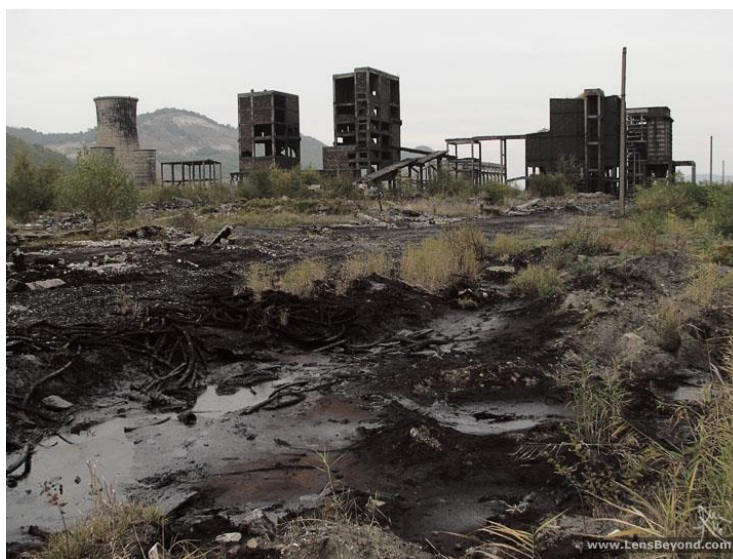
Figure 1: Abandoned site of the carbon-black factory in Copsa-Mica 18
